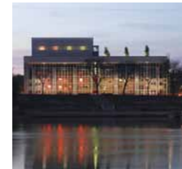
LE QUAI FACE À LA MAINE © ARCHITECTURE STUDIO
